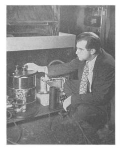
"TRINOSCOPE" — Heart of the RCA television receiver has three simple projection lenses through which images in red, blue and green appearing on three kinescopes beneath the lenses are projected in natural color on the screen at the top and front of the cabinet.
