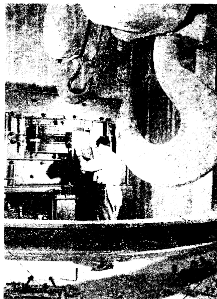
BETATRON —Exposure control ionization chamber is connected in the installation of the 20,000,000 volt betatron at the U. S. Army Arsenal at Picatinny.
