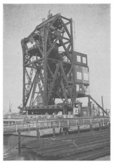
FLOATING CRANE—The largest self-propelled floating crane ever built is being readied by the Navy for Pacific waters. It is a jib-type of level-luffing construction. Its speed is 5.8 knots forward and 4.6 knots astern, and it can lift 350 tons 114 feet from its center of rotation.
