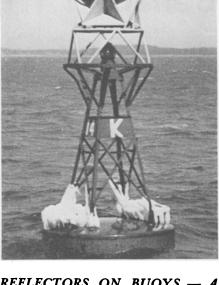
REFLECTORS ON BUOYS — A buoy wearing a radar reflector can be picked up by the ship's radar at twice the distance than when the buoy alone is the target.
