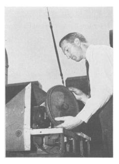
LIGHTNING HISTORIAN — Lightning writes its own history on the wheel of this "fulchronograph". Striking a tall mast, the lightning sets up an electric current which magnetizes small slices of steel inserted in the slots on the rim of the wheel. By measuring the amount of magnetism, engineers can determine the strength and duration of the thunderbolt.
