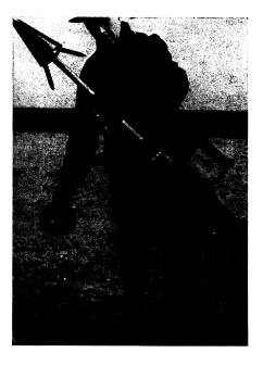
LIFE - SAVING EQUIPMENT — The backward projecting points on the line-carrying projectile anchor it in the ground when it strikes, giving a firm hold to the cable which has been unwound from the large reel shown.
