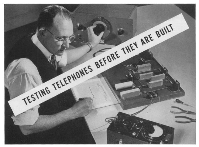
A TELEPHONE RECEIVER is a complex system of electrical and mechanical elements. Its coils, magnets, diaphragm and cap react on each other as they convert the electrical waves of your voice to sound waves. What is the best size for the holes in the ear cap? Will 1/1000th inch greater thickness help a receiver diaphragm to carry your telephone voice more clearly? One way to find out is to build numerous experimental receivers and test them.
