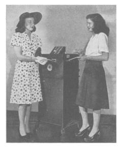
and issues a ticket to a passenger in an airplane station in less than five seconds. The machine in the picture, in a New York terminal, can issue tickets to cover at least 85% of the demands of travelers passing through the station.
