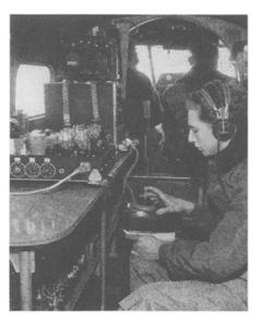
AUTOMATIC PILOT—This new, light-weight, all-electric pilot, normally mounted between the pilot and co-pilot, keeps the plane automatically on the radio beam. It was recently developed by the G-E Marine and Aeronautics Engineering Division for the Navy Bureau of Aeronautics.
