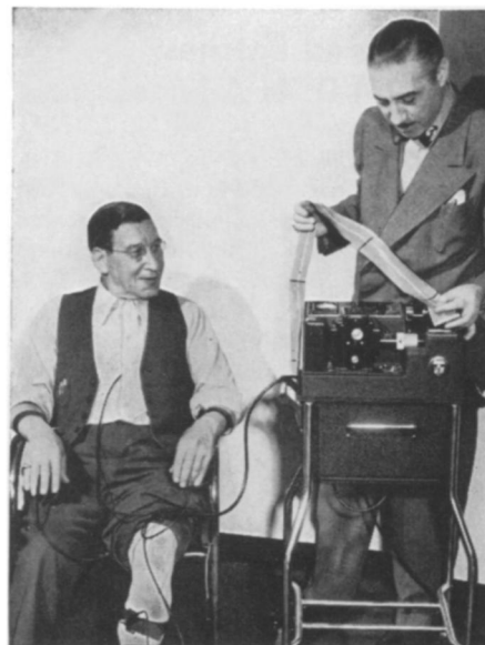
FOUR-SECOND CAMERA —The physician can read the record of a patient's heart almost as the beats are recorded. Shown at the camera is the inventor, Charles J. Glasser.
