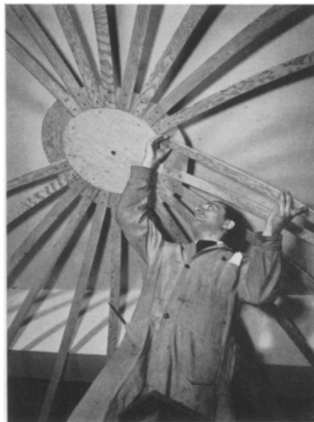
DOMES FOR SKY STUDY —Plywood ribs for the Penn State Dome are bolted to a circular piece of plywood as spokes are bolted to the hub of a wheel.
