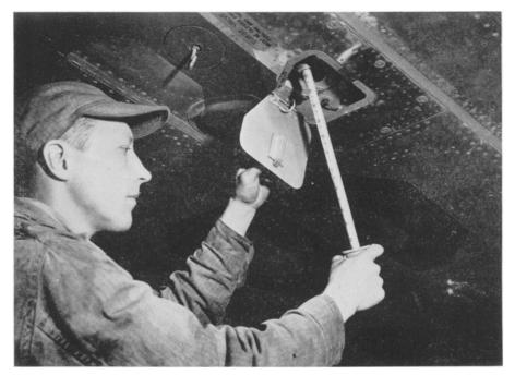
DIRECT READING GAUGE—Designed for use with the Martin 2-0-2's fast new under-wing fueling system, this gauge pulls down from inside the rubber fuel cell. A small ball, punctured with holes, on top of the gauge permits the fuel to trickle through the cylinder and drip out when the gauge reaches the level of gas in the cell. By reading the level at which it begins to drip, the mechanic can determine the fuel content.
