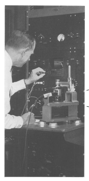
Your telephone receiver should treat each tone in the voice alike; that is important to you, because proper balance makes pleasant listening and easy understanding. Naturalness in receiver performance is pictured in a matter of seconds by the apparatus shown at left.
