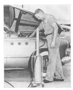
opening, thus eliminating the commonly used method of draining the tank from under the car. The 20-pound portable device, shown in the picture, works on ordinary air pressure.
