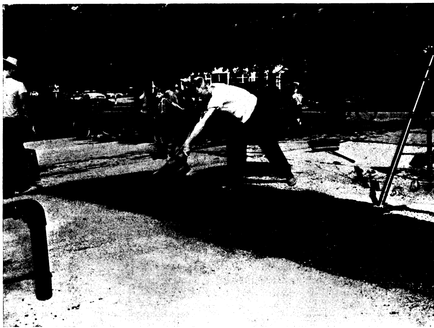
RUBBER-SURFACED PLAYGROUND —Ground-up rubber was mixed in asphalt for this test-installation of a new surface. It will mean a saving in shoe leather and clothing and will prevent skinned arms, legs and faces in accidental falls.
