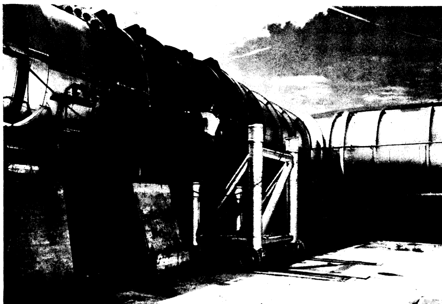
NEW SUPERSONIC TUNNEL —Most important single element of the huge tunnel is this 870,000 cfm axial flow compressor.
