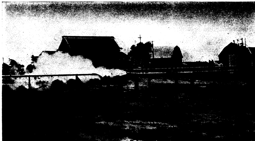
GASIFICATION TEST —Gas is escaping from the pipe sunk into the coal in the production of fuel gases from unmined coal by the use of electricity. This method eliminates the "cost of mining" factor.
