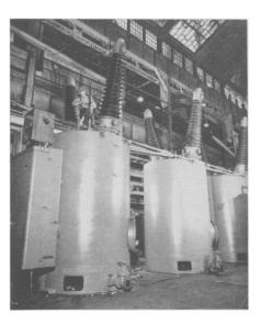
CIRCUIT BREAKER—The 10,000,000 kilovolt-ampere circuit breaker will assure hair trigger control of the tremendous electrical energy generated at Grand Coulee Dam. When the tanks are filled with oil, the giant assembly built by Westinghouse Electric Corporation will interrupt the flow of power in one-twentieth of a second.
