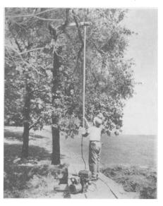
the ground. This electrically operated device, with pole removed, can be used as a hand saw. A small gasoline engine generator supplies energy, or household current can be used.
