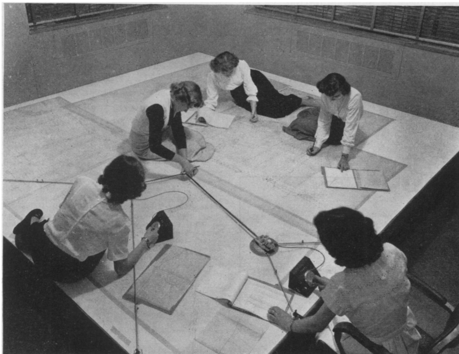
SEARCH FOR OIL-BEARING ROCKS —These women are plotting information gotten by magnetic surveys which will help Gulf geologists decide if a given area has prospects of being an oil producer.
