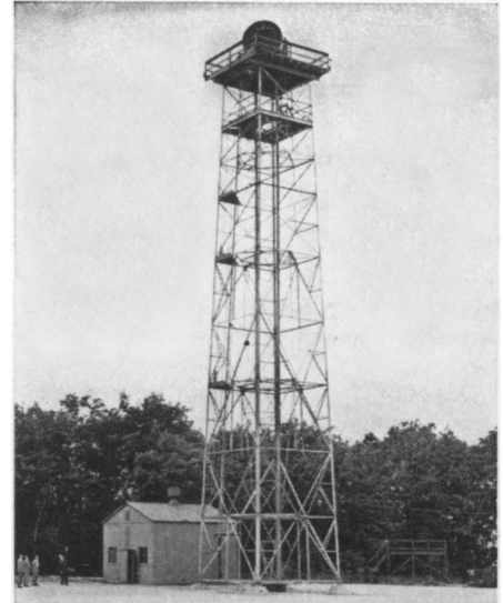
RADAR WEATHER TOWER— Advance storm warning is obtained by this detector at the Signal Corps Engineering Laboratories, Fort Monmouth, N. J.
