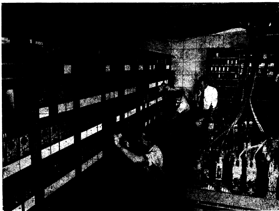
BEMAC COMPUTER —The entire computing portion of the BEMAC appears above with electronic components at left and mechanical section at right. Both sections are set up in "building block" fashion so that two or more relatively simple problems can be worked simultaneously.
