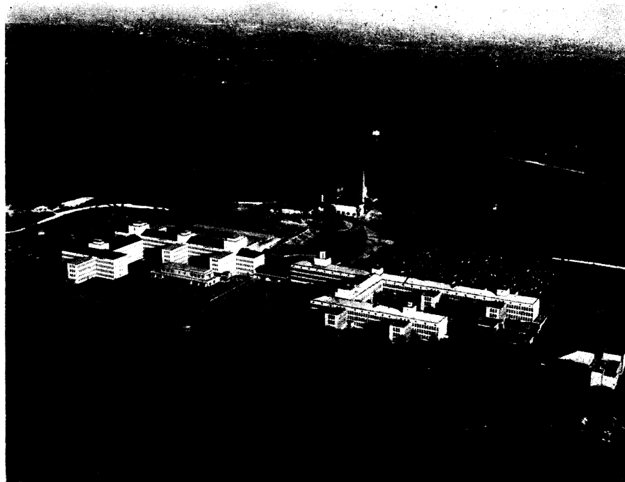
TELEPHONE RESEARCH HOME —The latest contributions of science and technology are applied to Bell System communications in the above laboratories. The country location about 25 miles from New York was selected to escape the noise, dust and vibration and electrical interference encountered in a metropolitan center. The acoustics building, containing the famous "dead room" is at the extreme lower right.
