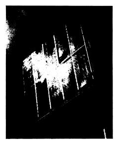
PLENTY OF BOUNCE—High-frequency radio waves or micro-waves strike this perforated aluminum reflector and bounce off at just the right angle to strike a receiving tower 12 miles distant. The sheet, which measures 20 feet square, is supported by a 50-foot tower erected on a mountain top.
