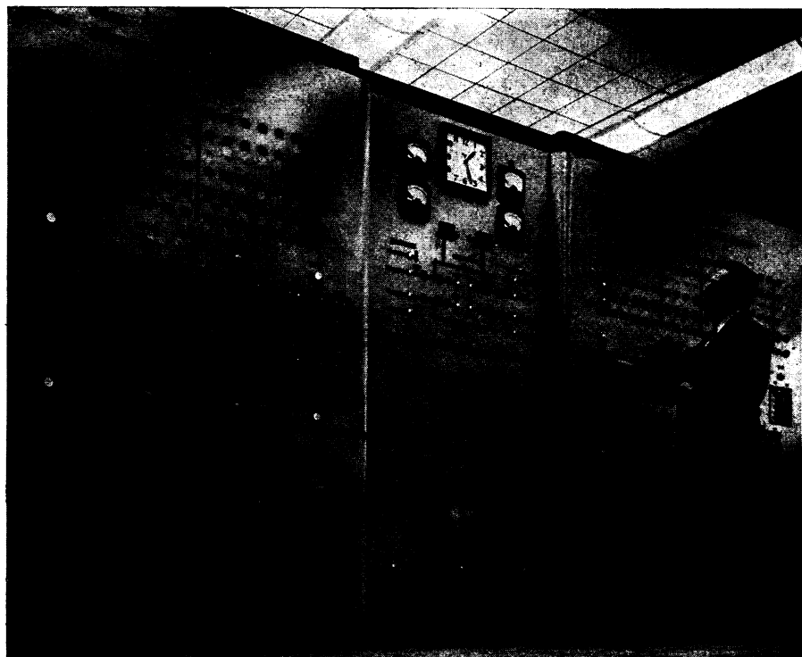
BROOKLYN BRAIN —The central brain of the new Brooklyn-Battery Tunnel's electric system controls ventilation according to carbon monoxide concentration. Carbon monoxide detector readings are continuously relayed to the control board, and flow of vehicles is regulated accordingly.
