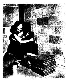
WONDERWALL, TWO IN ONE— The new Velon plastic wall panel not only insulates but decorates. Being applied directly over cinder block walls in the above picture, it can also be installed on wood, plaster, brick or concrete. The tongued and grooved edges make perfect fit and alignment
