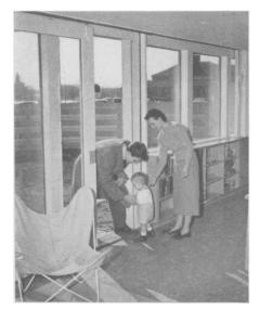
SUN WARMED—Large windows in the living room of the Massachusetts Institute of Technology solar house in Cambridge, Mass., help capture heat from the sun, but the main capture device is on the roof above. The heat storage tank containing water is just under the roof.
