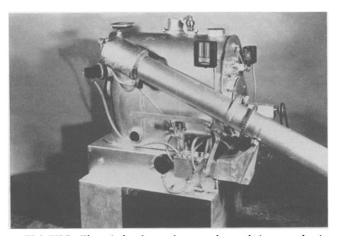
NEW STYLE—The unjacketed operating part of a revolutionary anthracite coal furnace reveals the tube in which combustion takes place. A stream of coal is fed into one end of the tube and air for combustion is drawn in the other end.
