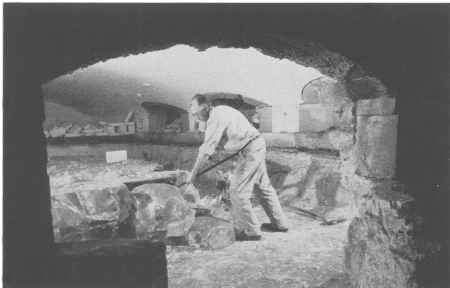
GIANT "GEMS" —This interior view of a glass furnace looks like a mine in which huge "gems" are being cut. Actually the worker is breaking away the solidified glass to permit maintenance work on the furnace walls, a task which must be done every 30 months.
