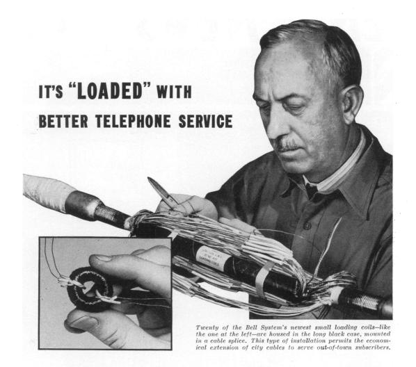
Many more wires can be crowded into a cable sheath when the wires are fine. But normally, wires don't transmit as well when they are fine and closely packed.
