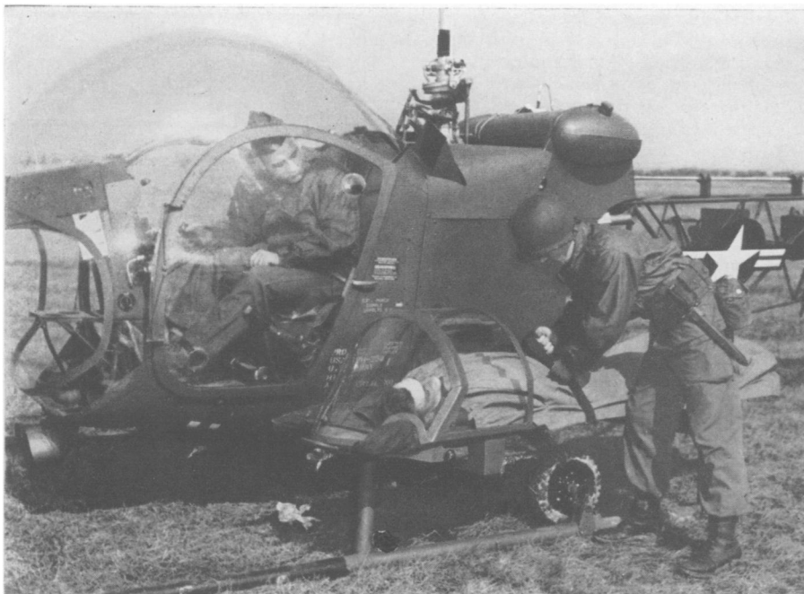
LITTER-CARRIER —For use in evacuating wounded from the battlefield, this Bell developed litter-carrier can be attached to the skid landing of a helicopter. It is designed to replace the troop-designed canvas "coffin-type" carrier used by troops in Korea.
