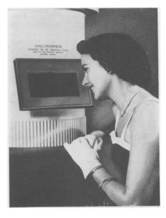
SPECTROSPHERE" is a cylindrical chamber with a viewing window, as shown in the illustration, used to compare the brilliance and fire of gem stones, the presence of single or double refraction and varia-
