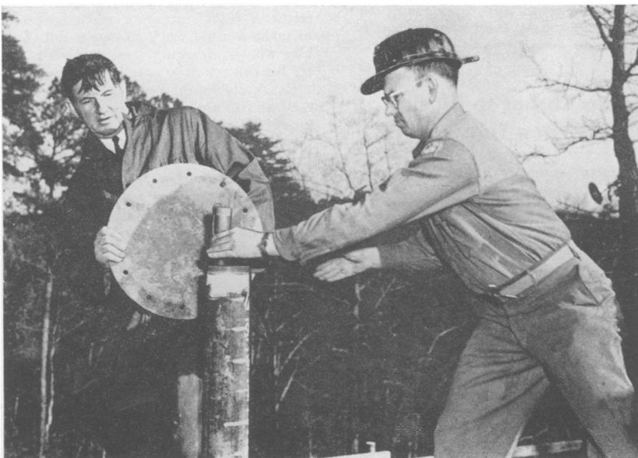
**COMBUSTION'S START**—An incendiary bomb, called a thermite grenade, is being tossed down a borehole to start combustion by U. S. Bureau of Mines' men in the second coal-gasification experiment at Gorgas, Ala.
