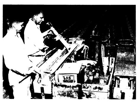
FERTILIZER USE—The best way to place fertilizer is being learned through studies such as this, where radioactively tagged fertilizer, loaded on an endless belt of hoppers, is distributed to a field. One scientist is checking the radioactivity hazard as the "hot" material is poured out through the metal tube.
