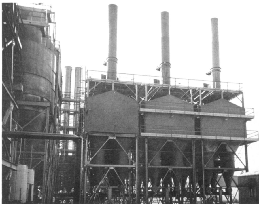
SOOT CATCHER —Last traces of carbon black are removed from the flue gas in these three bag filters where the soot-carrying gas is passed through the finest Orlon fabric. Note that no soot escapes from the stacks.
