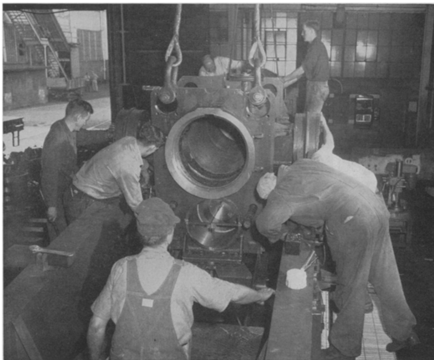
NEW WEAPON —This new gun for atomic missiles is being assembled at the Dravo Corporation's Pittsburgh plant. The cradle for the barrel is here being assembled to the carriage.
