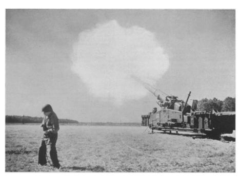
ATOMIC CANNON—This is the U. S. Army's newest weapon, the 280-mm. gun which is capable of firing either conventional or atomic shells. Here it is firing a conventional shell in a demonstration at Aberdeen Proving Ground. The gunner at the left, standing about 75 feet from the gun and with his back turned for protection from the blast, has just fired the gun by twisting the handle on the firing key.
