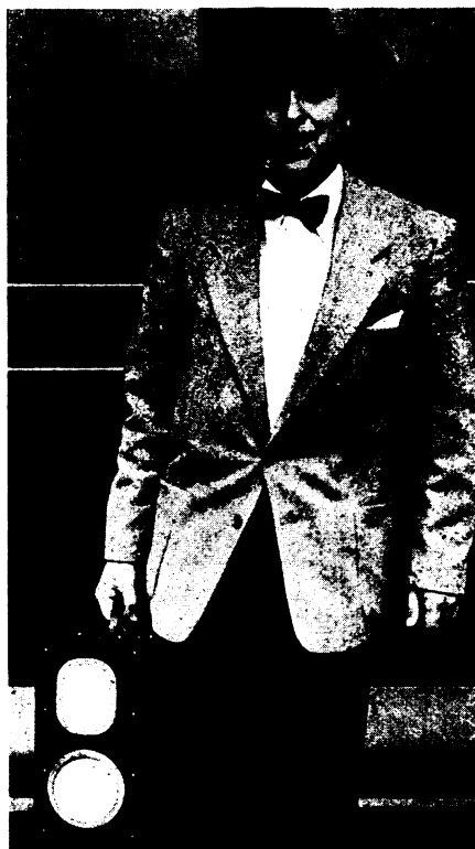
PORTABLE TV VIEWER —George C. Sziklai of the David Sarnoff Research Center at Princeton, N. J., carries an experimental battery-operated TV receiver. The set, weighing only 27 pounds, uses transistors entirely, except for the five-inch kinescope picture tube.
