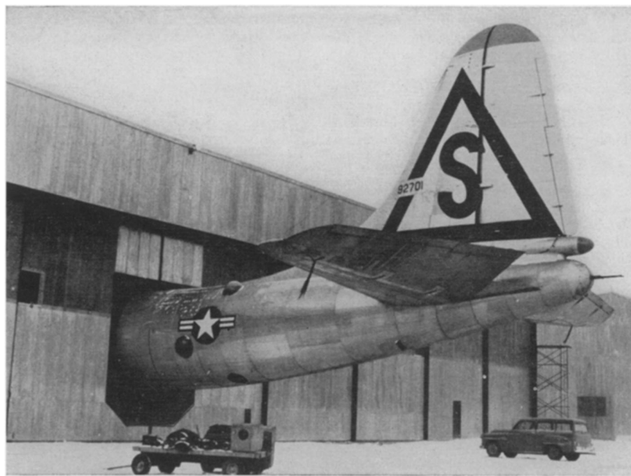
ALL-WEATHER BOMBER MAINTENANCE —New standardized, all-weather maintenance hangars for B-36's, designed by Luria Engineering Company, incorporate special features to enable U. S. Air Force personnel to perform around-the-clock repairs. The bomber's tail protrudes through a rubberized-tube door opening, which, when inflated, provides weather-tight protection around the fuselage.
