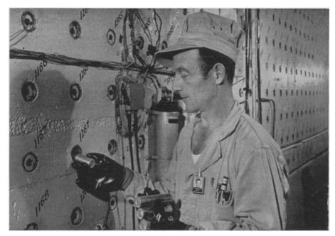
LOADING URANIUM SLUGS—Ten pounds of the precious fissionable material are being put into the holes of an atomic reactor at the Oak Ridge National Laboratory of the Atomic Energy Commission. Openings in the shield are round, but each channel in the graphite cube itself is diamond shaped, giving a passage for cooling air. From such an atomic power producer come radiations that are being used in a variety of promising ways.
