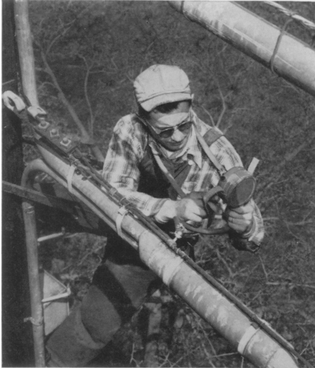
Air compressor and tank are at right. Long cylinders on rack dry air before it enters cables.
