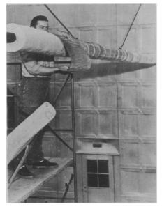
It is held in place with staples, adhesives or cords, and is jacketed in roofing felt, white asbestos paper-faced felt or thin sheets of metal.
