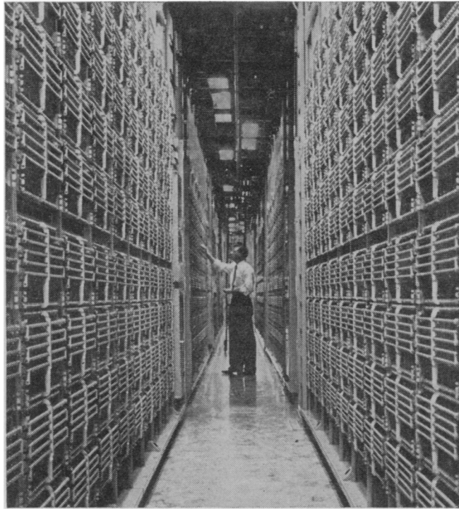
In a large, modern telephone office, two million relay contacts await the orders of your dial. They open and close a billion times a day.
