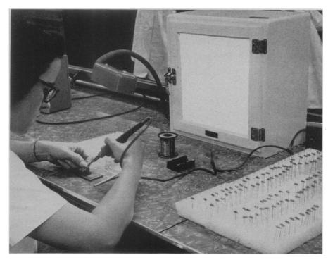
MORE EFFICIENT TRANSISTORS—Newest entries in the transistor field are "tetrodes" and "pentodes." They have three and four wires, respectively, running from the germanium nugget, instead of two, and can do the work of two or three of the triodes shown here during assembly.
