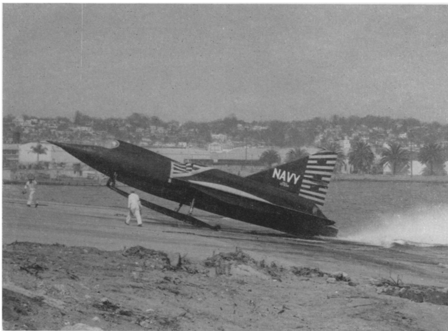
NAVY'S SEA-DART—The first combat-type aircraft to use water skis for improved rough water take-off and landing operations is the Navy's XF2Y-1 Sea-Dart, experimental delta-wing jet fighter shown here. Retracted, the hydro-skis disappear into the hull to give the plane a missile-like look. (See SNL, Jan. 3, p. 6.)
