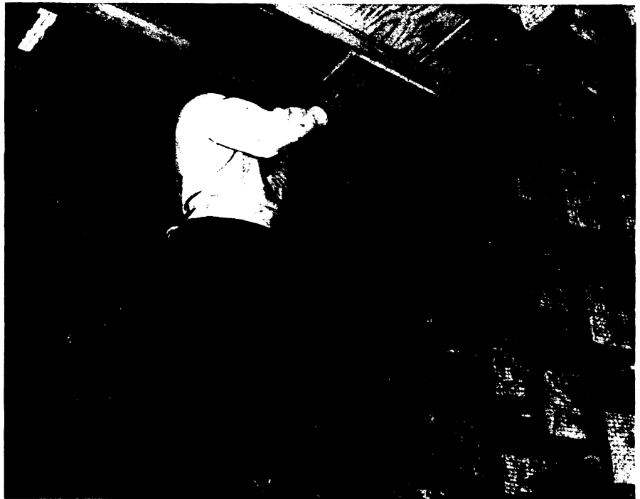
SILENCE MADE-TO-ORDER —Sound absorbing wedges of glass wool are installed in a new echo-free chamber at Indiana University by Prof. James P. Egan of the psychology department. Completely lining the room, they will "soak up" all but a thousandth part of sound striking them.
