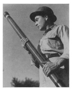
impractical. Made of rugged butyrate plastic, this new screen, shown in the photograph, does not shatter or corrode, resists most oils and greases, comes in lightweight, five-foot sections in diameters up to four inches, and is said to be ideal for wells up to 200 feet deep.
