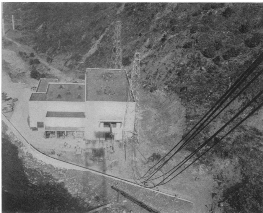
"BIG JIM" RADIO STATION —Looped in giant strands across Jim Creek Valley, Arlington, Wash., 150,000 feet of steel copperweld cable form the largest radio antenna ever constructed. This is a bird's-eye view through the steel framework of a 200-foot summit ridge tower showing the transmitter building in the valley between 3,000-foot mountains. Special precautions have been taken to protect personnel from the invisible but dangerous energy at the most powerful radio station known to the Western world.
