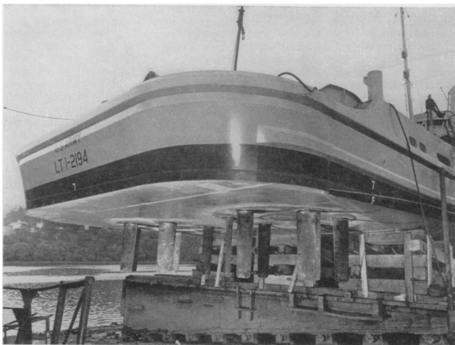
VERTICAL AXIS PROPELLERS —"Business ends" of the vertical axis propellers on the rudderless tugboat are these blades, each four and a half feet long, that project downward from the stern.
