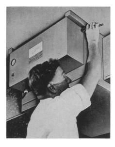
ing, as shown in the photograph. Attached to the main return air duct of a forced-air heating system, the device screens 90% of all airborne dust, pollen and tobacco smoke particles from an average five- to seven-room house. It has no moving parts.
