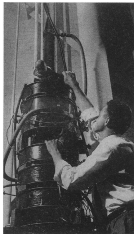
GIANT KLYSTRON —First photo of the 4,000,000-watt klystron designed to power an advanced Air Force radar. The eight-foot giant, prototype for a series of the military's most powerful microwave tubes, is shown undergoing installation in a high-power radar transmitter room at Griffiss Air Force Base, N. Y.
